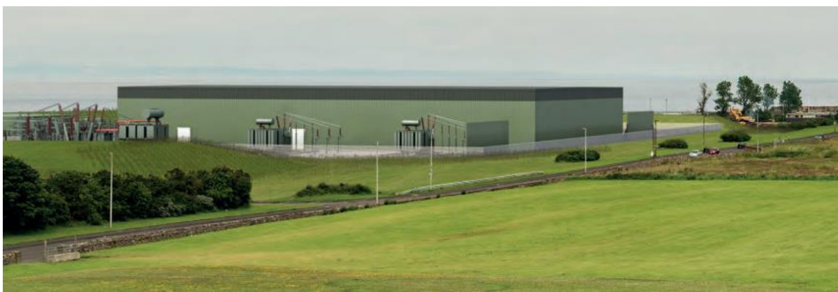
ICOL Building type photomontage looking from bund to the south west at 380m distance (image to be updated when available)
